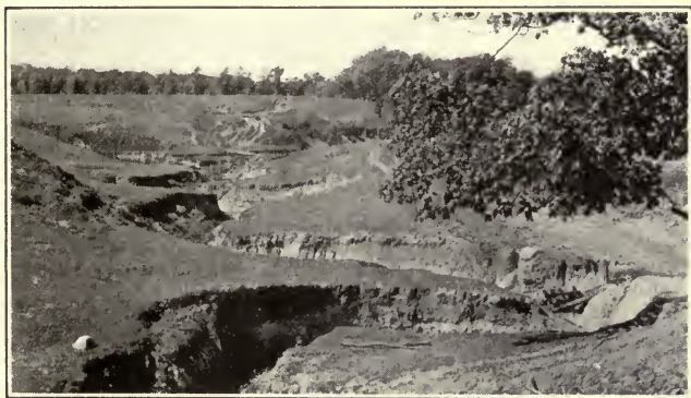
DAMAGE BY EROSION
